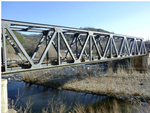
Figure: Truss Bridge
